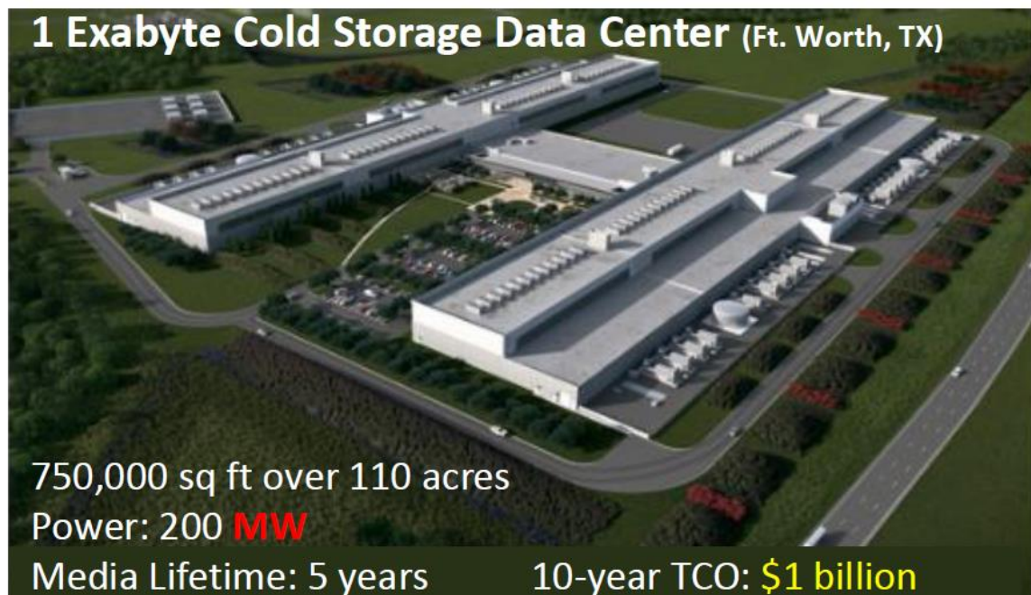
Figure 1. Example of the physical requirements of hyperscale data centers. Source: IARPA [1]
